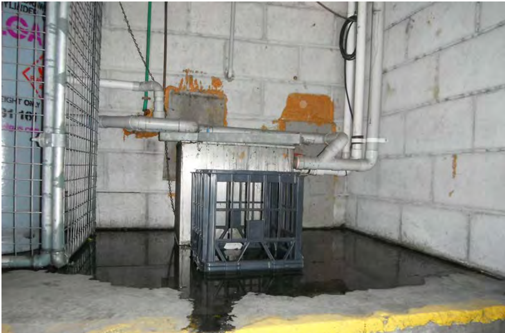
Photo 2 – Waste water filter system overflowing located adjacent to the LPG gas cylinders
